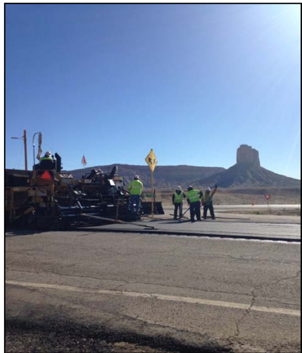
Leveling course paving at US 160/141 intersection
